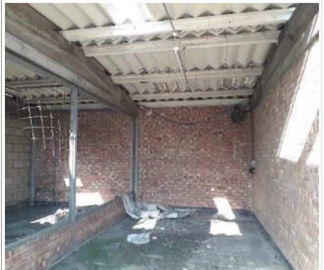
Photograph 4 – Internal of building 6
